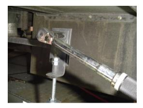
14. Tighten the outside top 5/16" nuts to the brackets. Keeping the hanger perpendicular to the ground. Torque to 9 ft. pounds.
