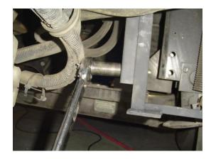
9. Tighten the bottom bracket to the top bracket. Torque bolts to 110 ft. pounds.
